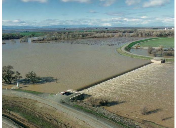
Figure 3, Moulton Weir, January 1997
