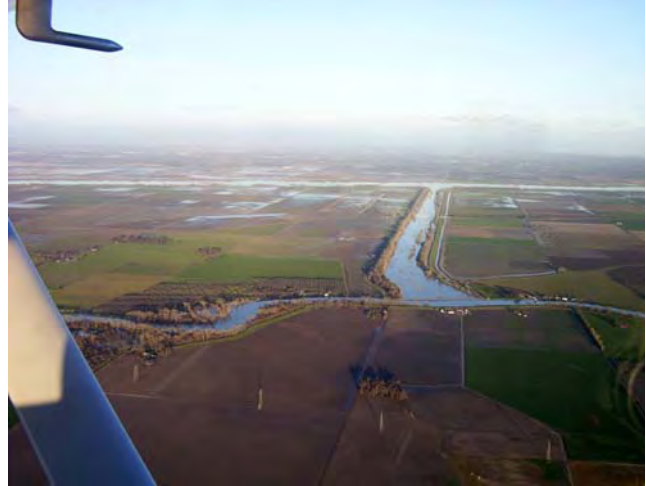
Figure 5, Tisdale Weir and Tisdale Bypass (Sutter Bypass in background, January 1997)
